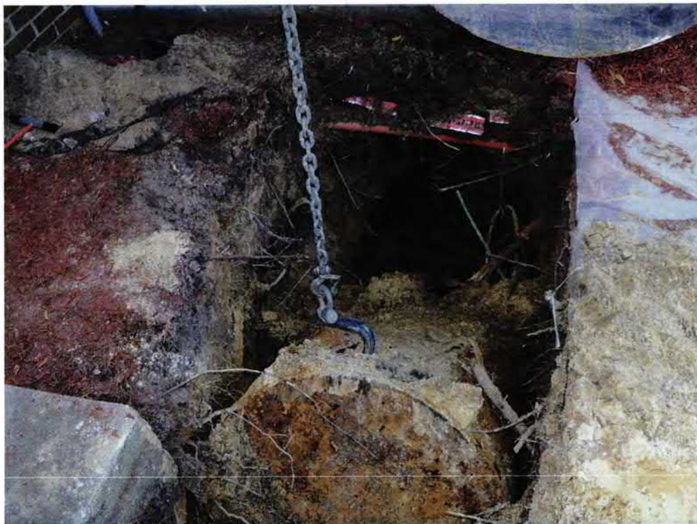
Picture 2: UST 361Aspen during removal.
